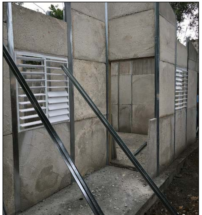
House slabs assembled like Lego pieces.
